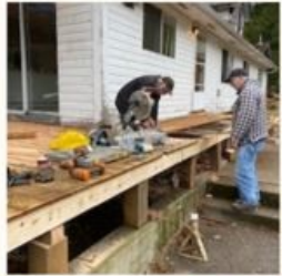
Lions working on the new deck for the caretaker's house.
